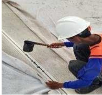
**Gambar 3.17** *Joint Sealant*
