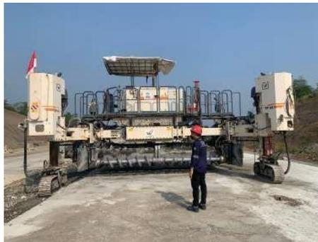
**Gambar 3.4 Concrete Paver**
